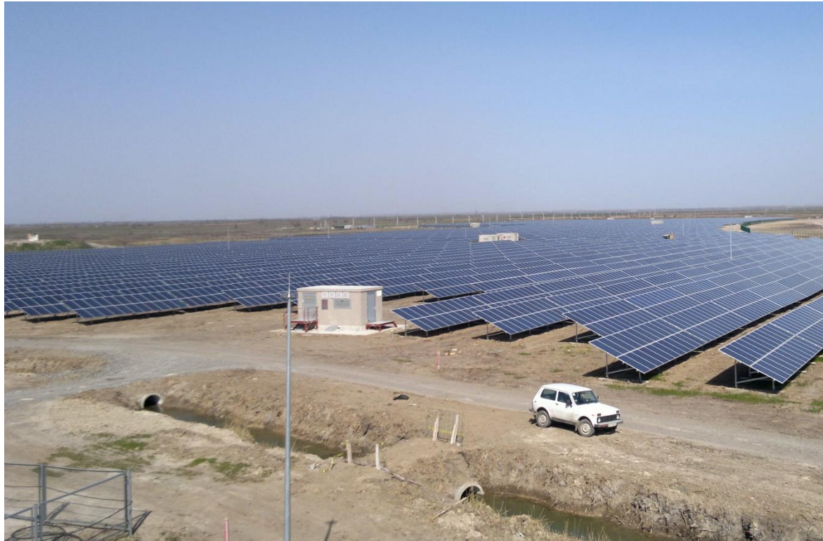
ESE lightning rod in a free-standing pole
