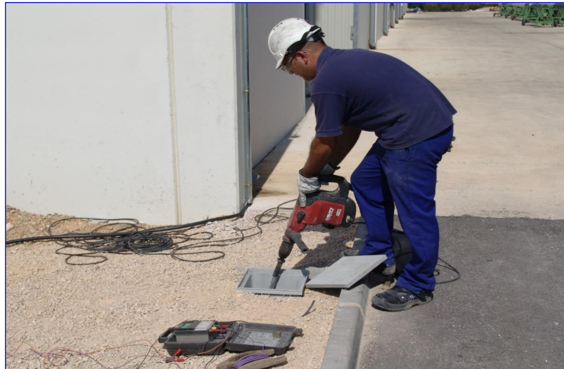
Installation of earth rods using an electric hammer
