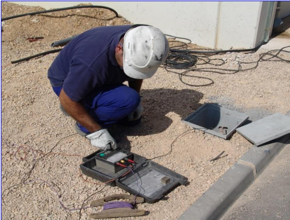
Measurement of an earthing system with 2 references
