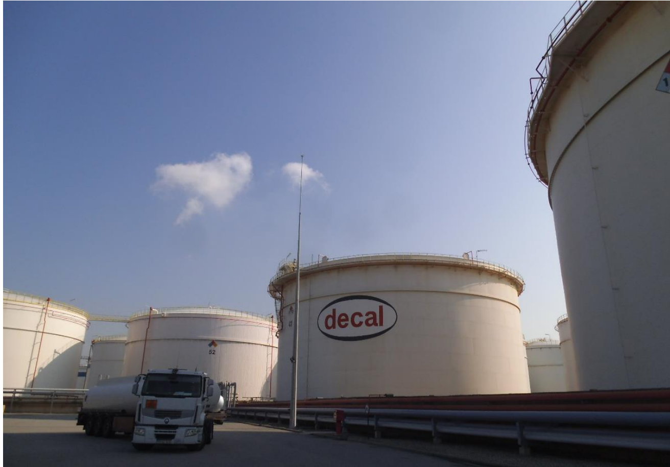
Lightning rod in a free-standing pole
